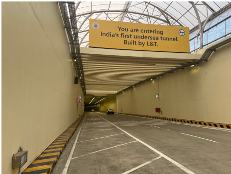
Mumbai Coastal Road Tunnel
