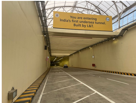
Mumbai Coastal Road Tunnel
